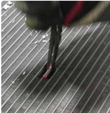
Figure 15. Crimp the aluminium wrapper with needle nose pliers
