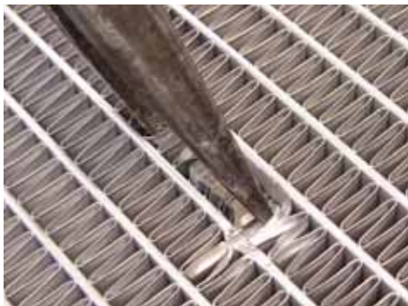
Figure 10. Clear away approximately 1" of fin material
