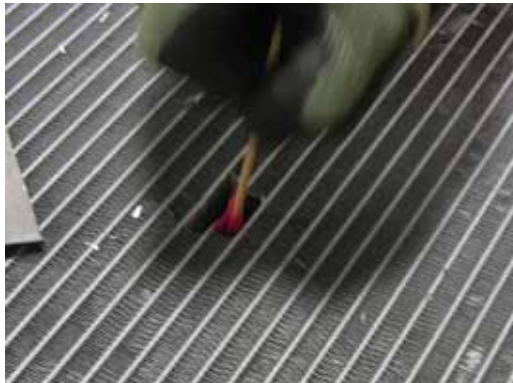
Figure 12. Apply epoxy to the leaky area
