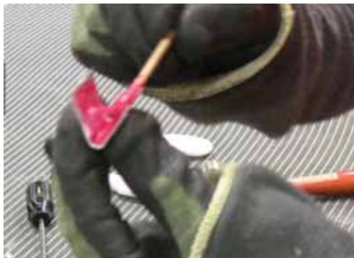
Figure 13. Apply epoxy to the aluminum wrapper
